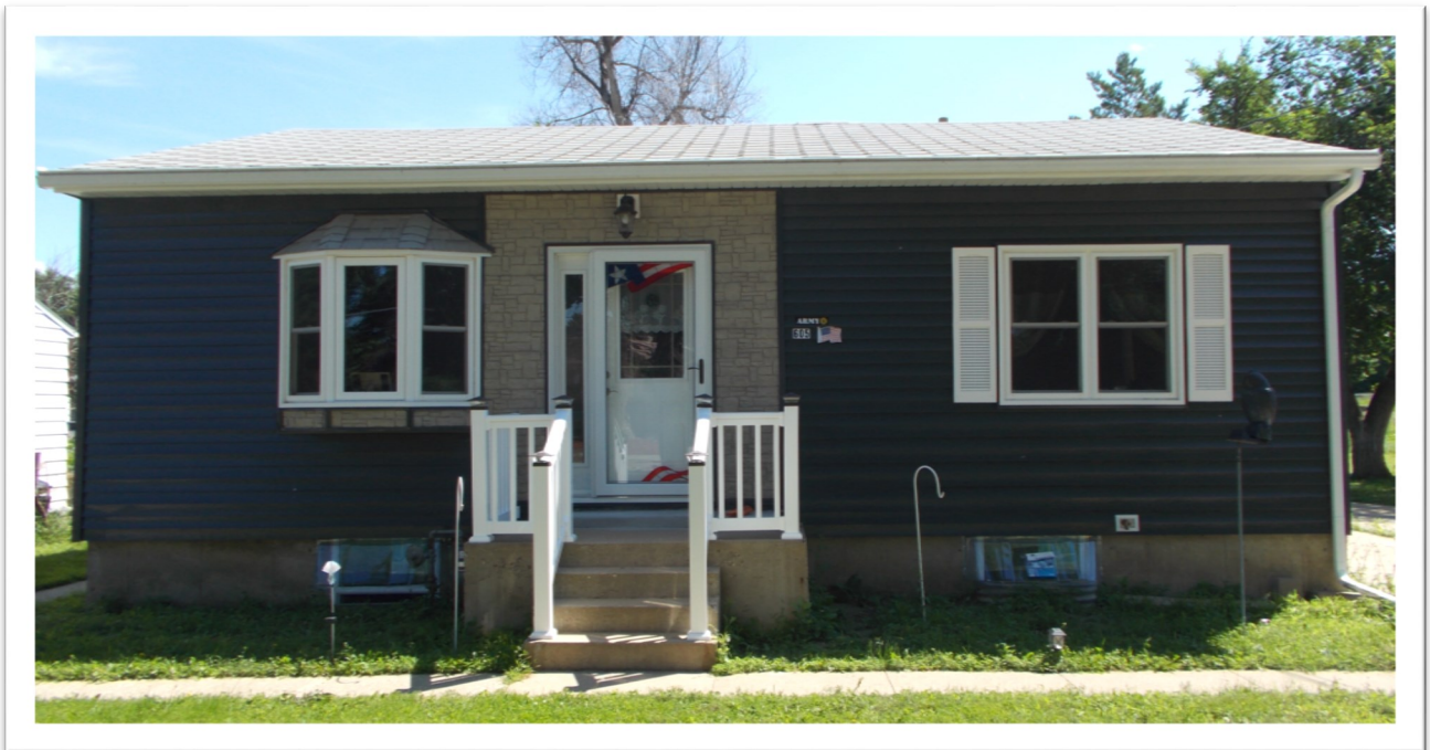
A home rehabilitated by DSW Homes in Minot, ND.
