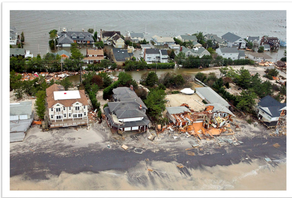
Damage along the New Jersey coastline from Hurricane Sandy.
