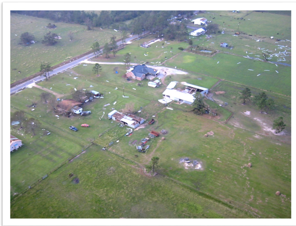
Damage as a result of Hurricane Rita
